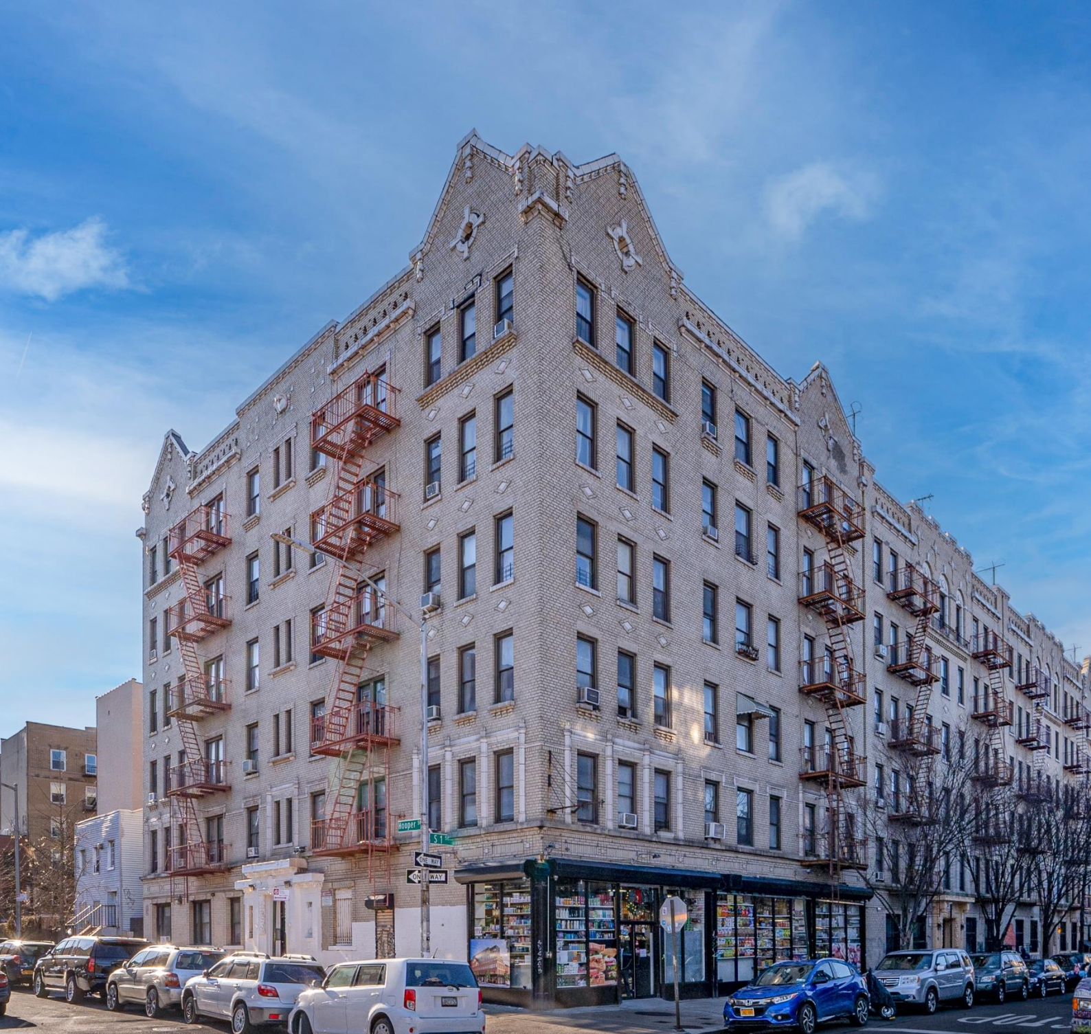
Residential Building in Brooklyn, NYC
